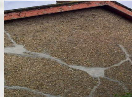
Image taken from a house near Camborne showing irregular branching cracks (many recently repaired) in render overlying seriously degraded blockwork. The aggregate is a sulfide-rich copper-arsenic mining waste typical of the northern part of the Camborne - Redruth mineralised district.
